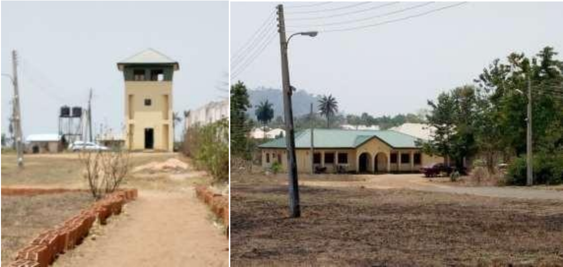
Some of the Prison's infrastructures.
