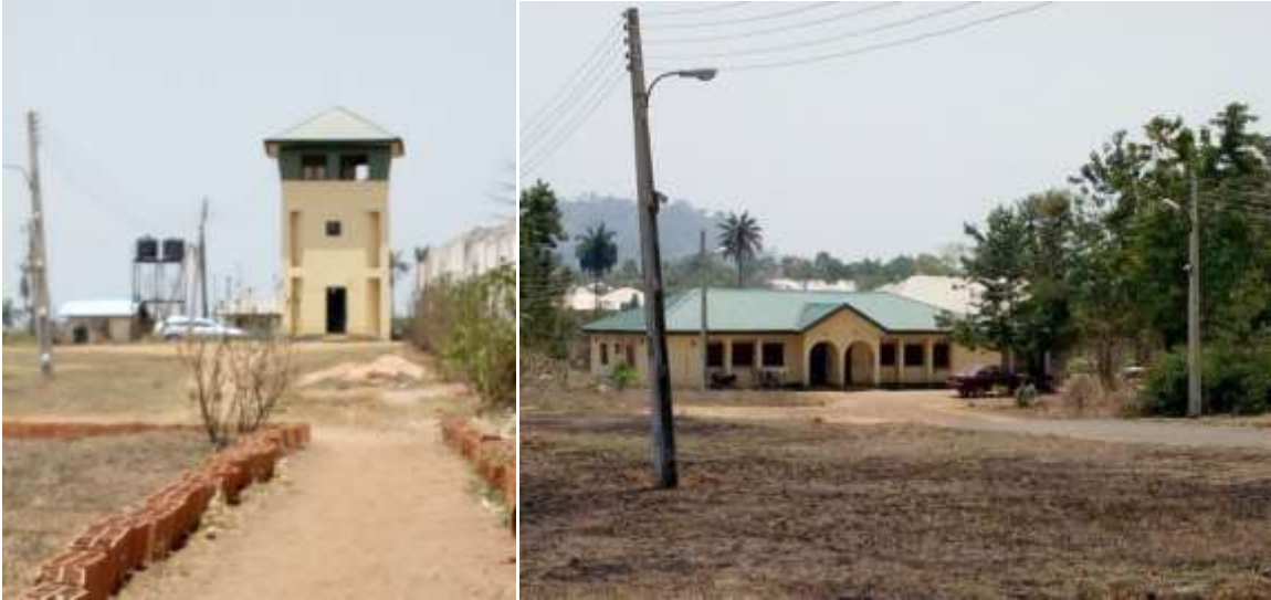
Some of the Prison's infrastructures.
