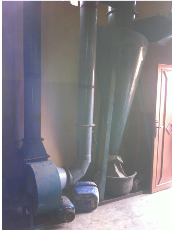
The compressor unit of the pelletizing machine
