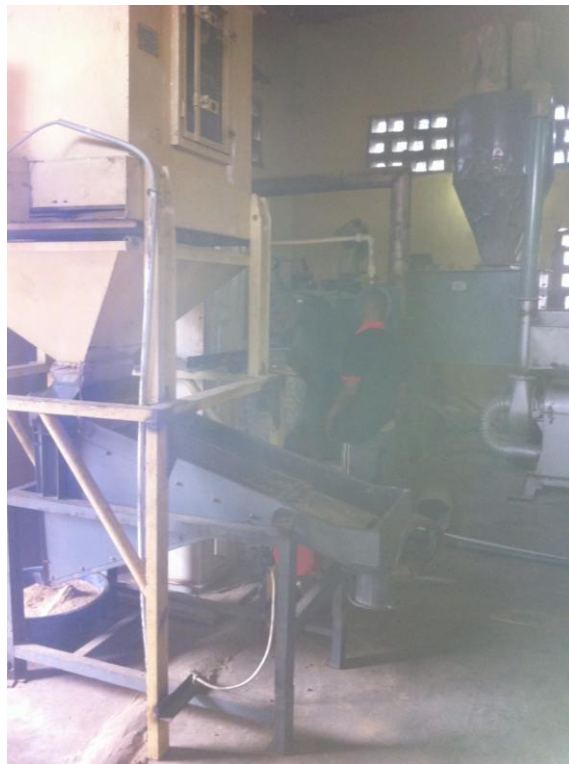
A combined pellet milling machine (hammer mills and vertical mixer)
